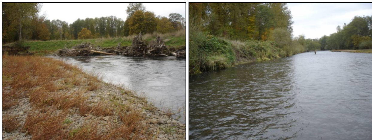
Figure 4-8. Examples of bank stabilization in Reach 3 include the Ross site (left) and an older riprap project spanning 2,000 ft from Sta. 242+00 to 262+00 (right).
