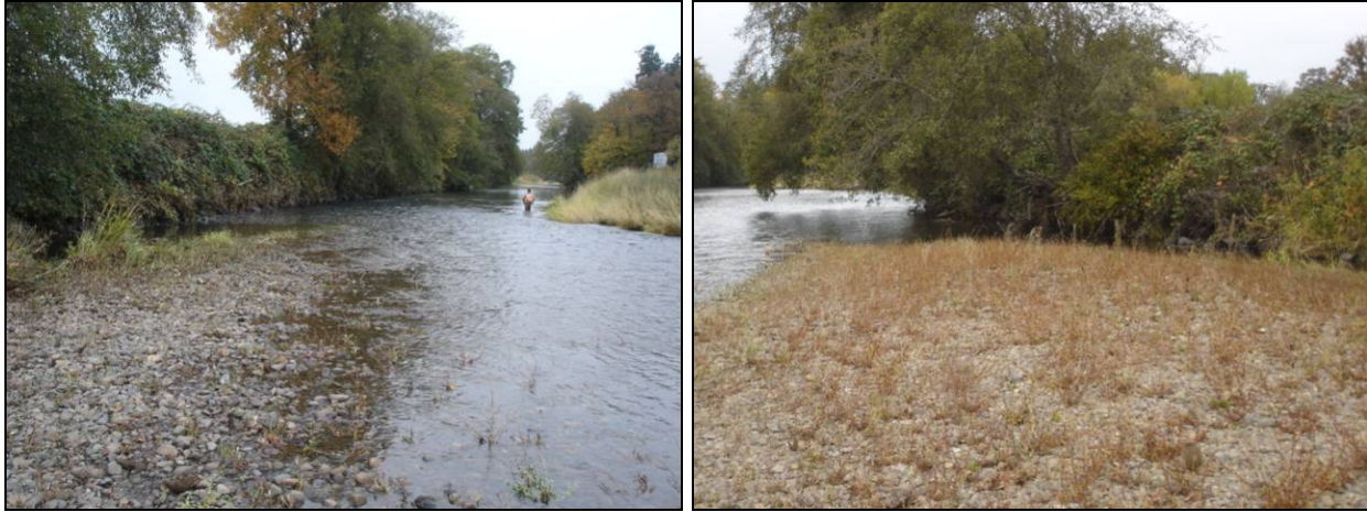
Figure 4-12. Examples of bank stabilization in Reach 4. The left bank is stabilized in upper Reach 4 (left). Blackberry bushes and deciduous trees have colonized the riprap. The right photograph shows a backwater habitat that has formed between a gravel bar and the adjacent riprap bank at station 309+00.
