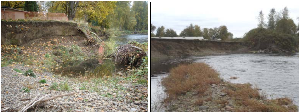
Figure 4-9. The bank erosion site downstream from Pioneer Park that continues onto the Gerber and Smith properties (left), and the vertical streambank on the Nealon property (right). The blackberry covered structure in the middle of the right photograph is a rock spur or levee.
