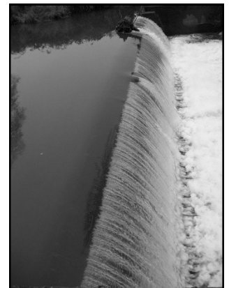
Sodom Dam, photo CWC 2009.
