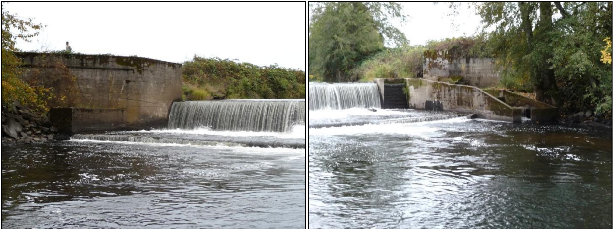
Figure 4-4. The river-right abutment that will be lowered to provide access to the dam apron will also be removed as part of the project (left). The fishway on river-left will be used for fish passage and clear water bypass during dam deconstruction (right). The fishway and river-left abutment will also be removed.
