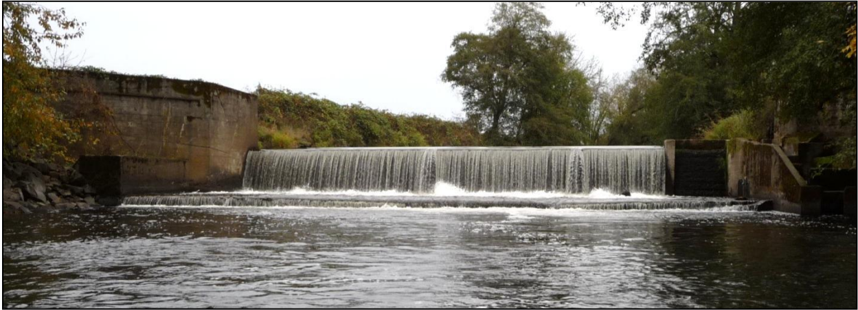
Figure 4-3. An upstream view of Sodom Dam showing the river-right abutment, dam face, the portioning wall between the dam face and river-left fishway, and the river-left fishway.
