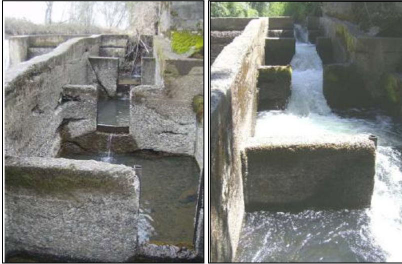
Figure 7-1. The Sodom Dam fishway. The left photo shows the ladder when the upstream inlet is plugged with debris. The river photo shows the ladder under operational conditions. Photos courtesy Crispin (2010).
