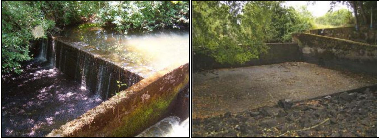
Figure 7-3. Shearer Dam on the Calapooia River under low flow (left) and dry (right) conditions. Coarse bed material located downstream from the dam is believed to be remnant material from the historical timber crib dam that preceded the existing concrete dam. Round rock will be imported to provide near-term streambed stability once the dam is removed. Photos courtesy Crispin (2010).
