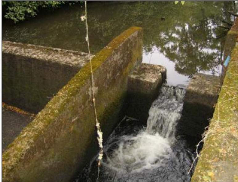
Figure 7-2. The Shearer Dam fishway inlet. The fishway is of similar pool-notch construction as the Sodom Dam fishway. Photo courtesy Crispin (2010).
