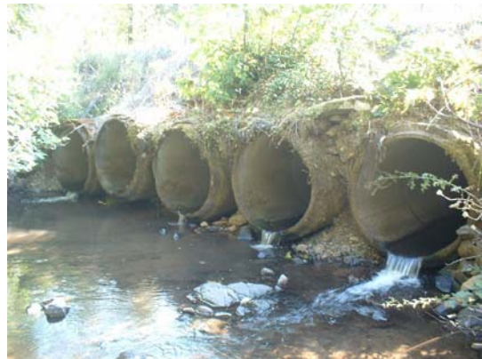
Reach 2 - Unit 187 5 Culverts in a row
