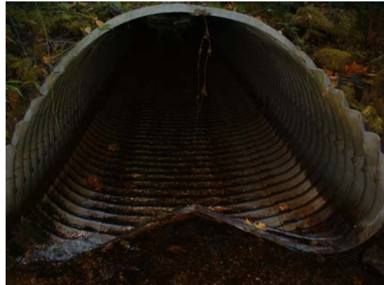
Reach 2 - Unit 208 Culvert - The end is crushed
