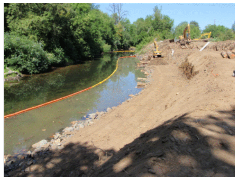
EXAMPLE OF FLOATING SILT CURTAIN PLACEMENT
