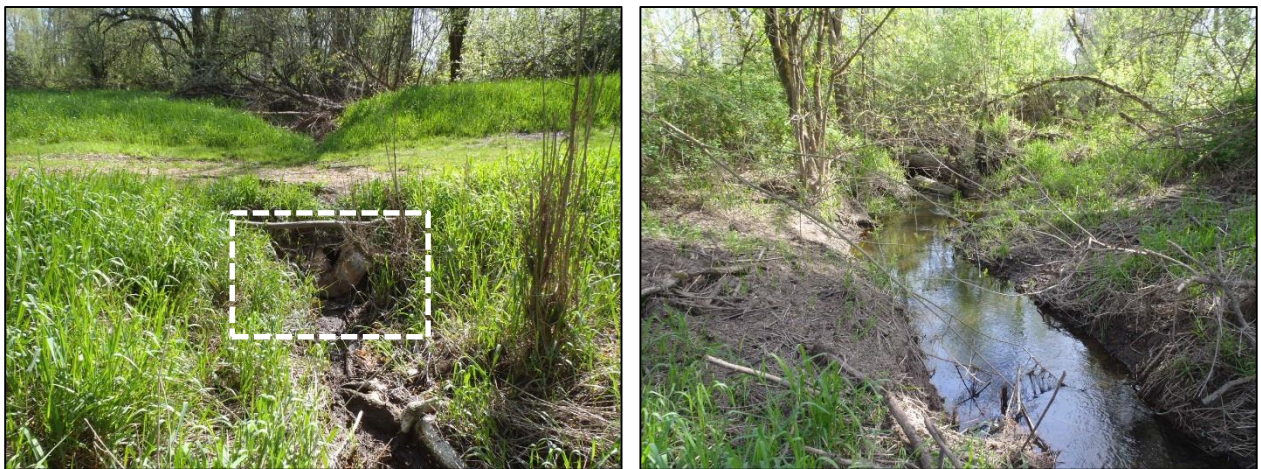
Figure 4-11. A downstream view of WS-3 (left) showing the minimal road fill over the culvert (white box), and a downstream view in the West Slough towards the East Slough-East Slough confluence (right).
