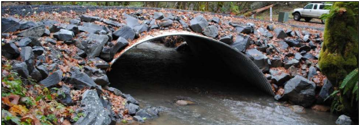
Figure 6-4. View of an open-bottom arch culvert with installed streambed.
