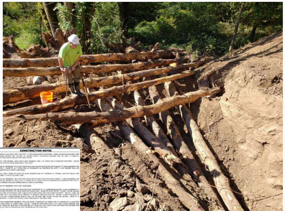
All thread rods installed between each tier of logs
