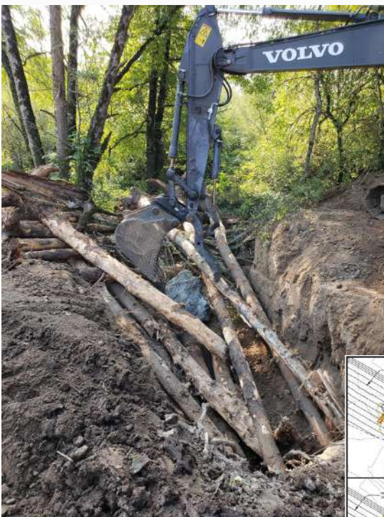
25 ballast boulders placed on logs
